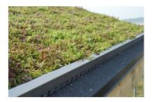
**5.** Cut edges are not allowed placed against the edge finish or against a leaf catcher with drainage holes.
