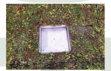
7. When installing against Nature Impact<sup>®</sup> Roof's leaf catcher, the modules must be placed all the way to the edge of the leaf catch. Rounded stones are <u>not</u> used between the leaf catch and modules, as this will reduce the drainage capacity.
