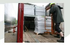
**1.** Upon receipt, the modules should be inspected. The wrap on the pallets should be removed at once after they are transferred to the roof.
