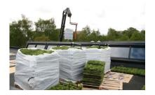
**2.** The installation must take place as soon as possible after receipt. No later than 48 hours after receipt.
