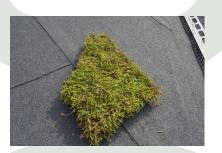
**4.** The modules are cut to size as needed, e.g. with large insulation knife. Cut against a cut-resistant substrate. Never cut directly against the membrane.
