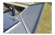
**8.** For valley gutterss and the like, a support profile is welded on to which the modules are laid up against.
