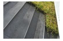
**6.** On roofs with a slope >15 degrees, support profiles must be welded on to prevent modules slipping. See diagram for mounting on pitched roofs.
